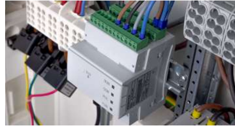
Fig. 42 ADW200 mounted on top-hat rail (DIN 35 mm)
